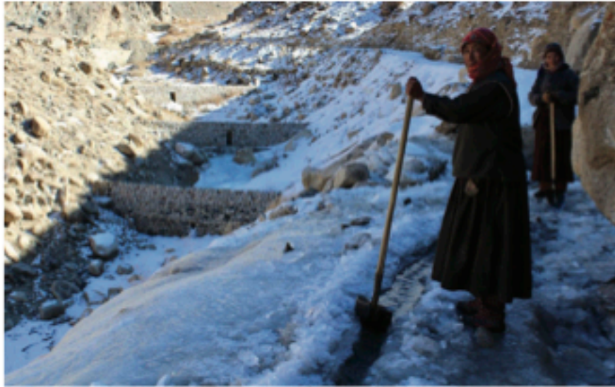
Figure 6. Villagers in Nang must break up ice in the diversion canal to their AG on a rotation basis throughout the winter Photo: Sierra Gladfelter (2017)
