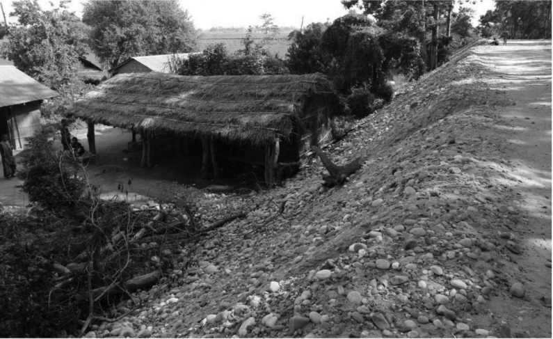
Image 6: A partially completed embankment built to protect this community on their land has also created everyday challenges for them including waterlogging in their fields, erosion of stone and sand that washes into their yards, and difficulties in accessing the road and river (Photo by author).
