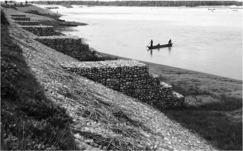
Image 1: This embankment was built during the Karnali River Training Project's first year of construction to deflect the river back toward Tikapur, directly across the river and from where this canoe ferry is coming (Photo by author).
