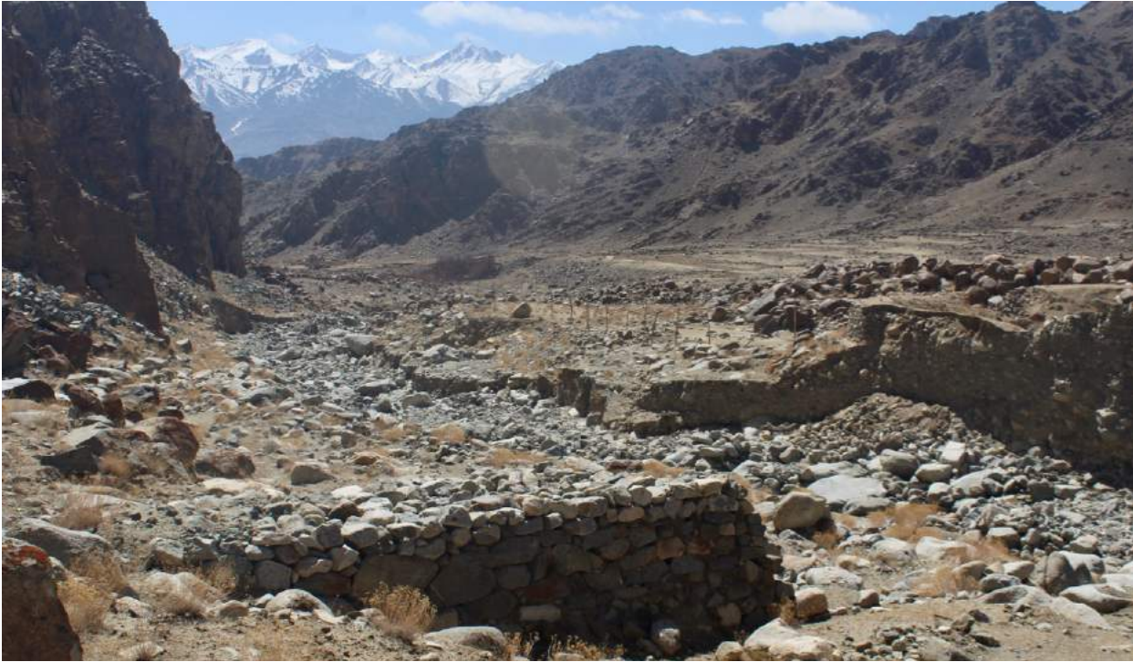
Figure 24. A downstream view of the damage to Stakmo's AG and scouring of the stream channel.
