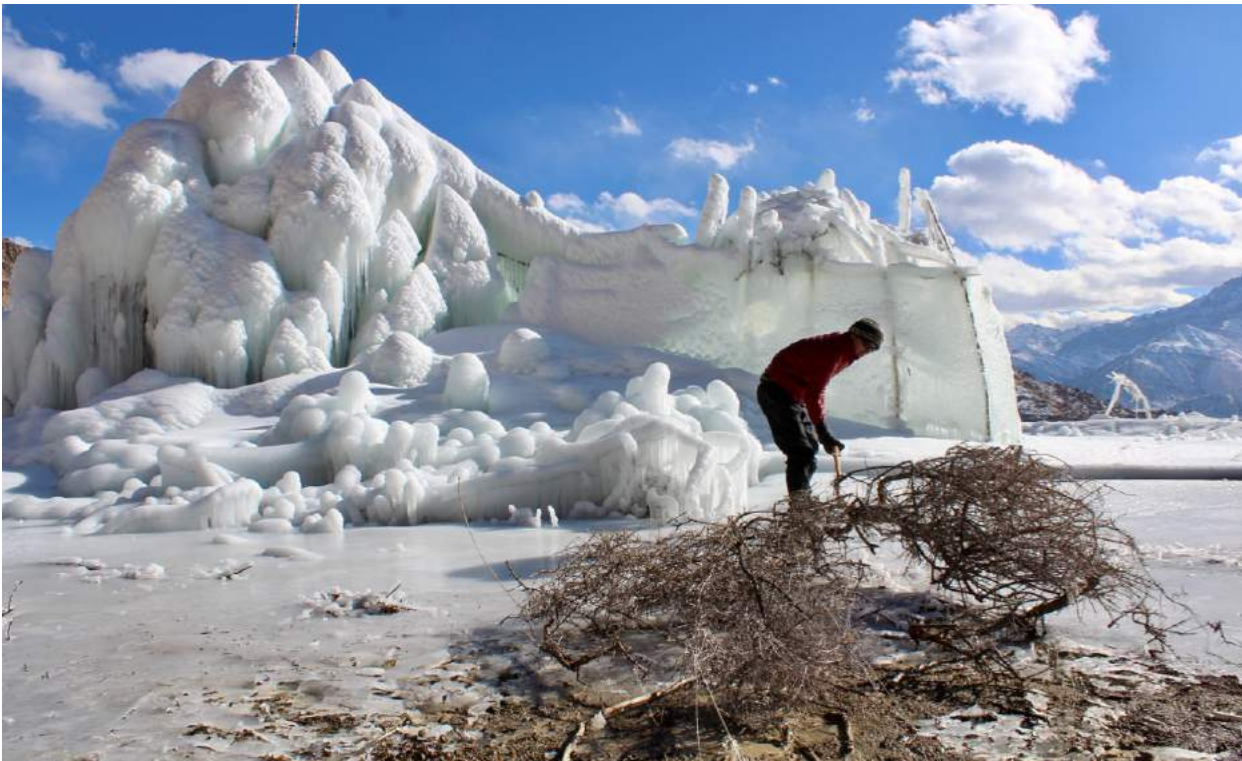
Figure 30. Local materials like thorny seabuckthorn accelerate ice formation as water coats it. Other materials that the IS team has experimented with to increase surface area of the base structure include netting, barbed wire and razor wire.
