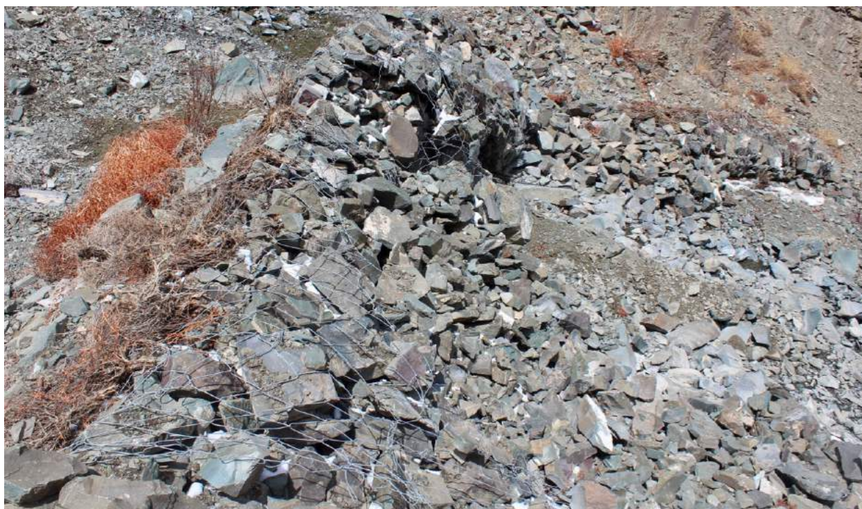
Figure 21. A broken wall at the AG above Takmachik, where summer flows in the stream channel rolled the entire wall downstream, shredding the crate wire and spilling out the rock contents.
