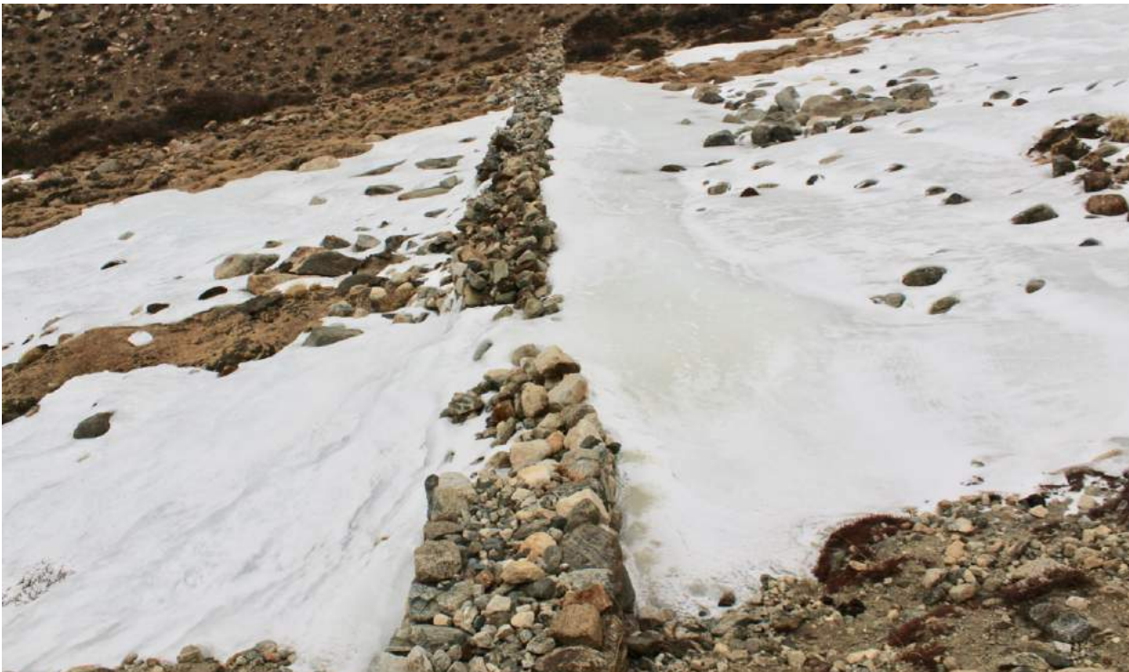
Figure 25. Although partially damaged, this wall continues to accumulate ice even at a fraction of its full capacity.
