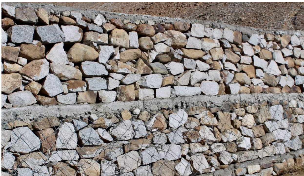
Figure 20. Double-layered stone, concrete and crate wire walls constructed at Likir in 2017 with Tata Trusts funds.
