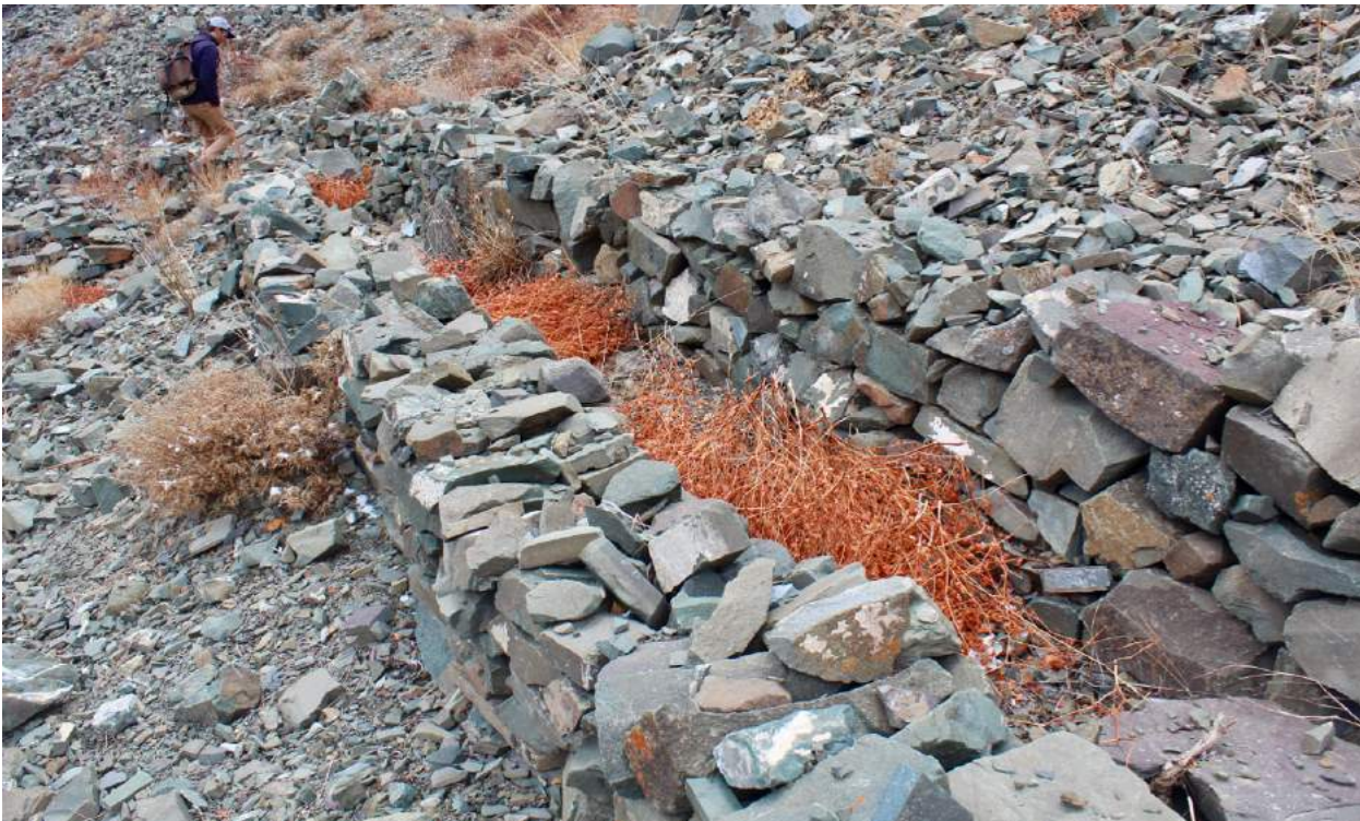
Figure 9. According to local residents, this diversion-style AG, built above Takmachik village, never functioned due to water loss through the loose stone and sand in this now abandoned diversion canal.
