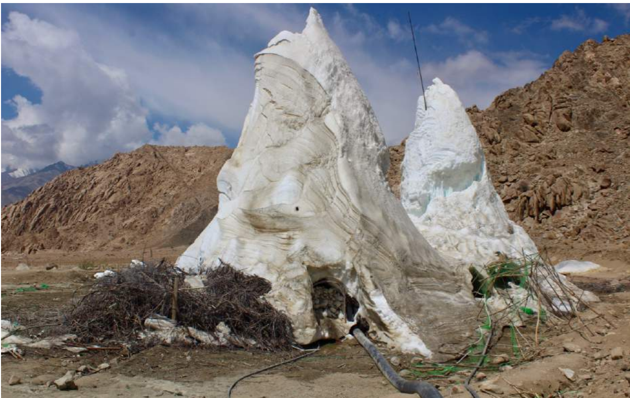
Figure 32. By early May, the IS has already melted considerably, revealing thick layers of ice.
