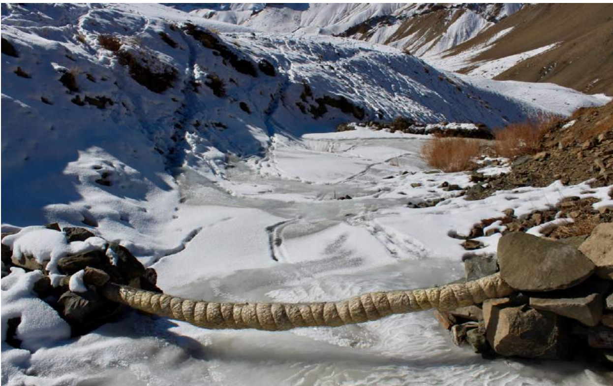
Figure 35. At all sites where AIGs have been built, pipes were buried to provide insulation and mitigate blockage. Here in Henisku where the pipe crosses a small stream, it has been wrapped in cloth and foam.
