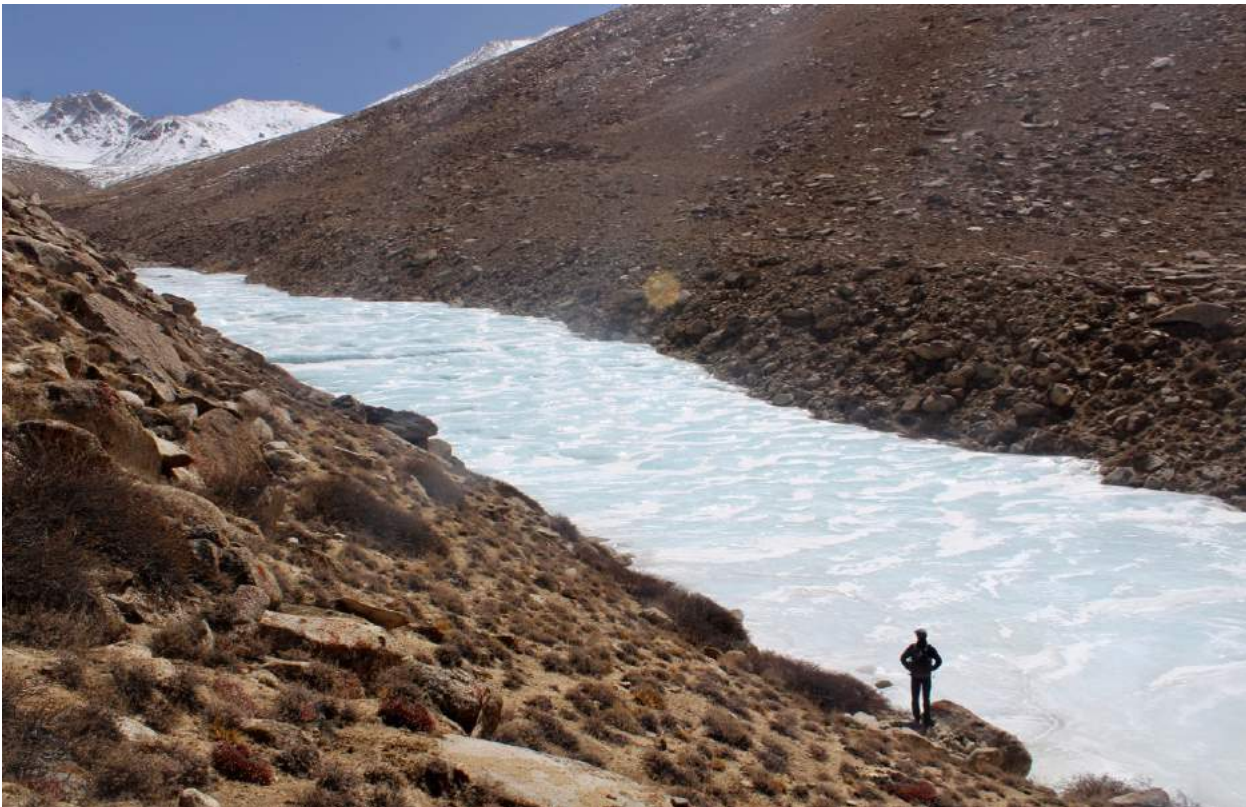
Figure 18. Igu village's AG built by the Leh Nutrition Project with support from the Tata Trusts. This structure has 24 walls and was built on top of traditional stone walls constructed by villagers over generations.
