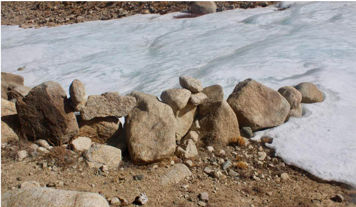
Figure 3. This is the remainder of a traditional single-stone wall at the site of the modern AG above Igu.
