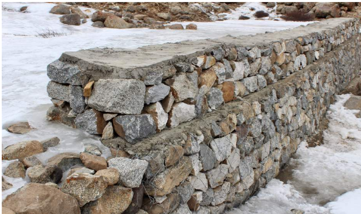
Figure 19. Recently constructed (fall 2017) concrete and crate wire-reinforced walls above Phuksey village.
