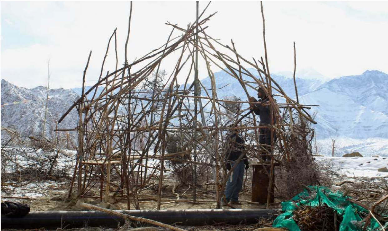
Figure 29. The first stage in construction is to build a frame which can support the initial structure until ice accumulation enables it to support its own weight. The hollow core also allows new sections of pipe to be added.
