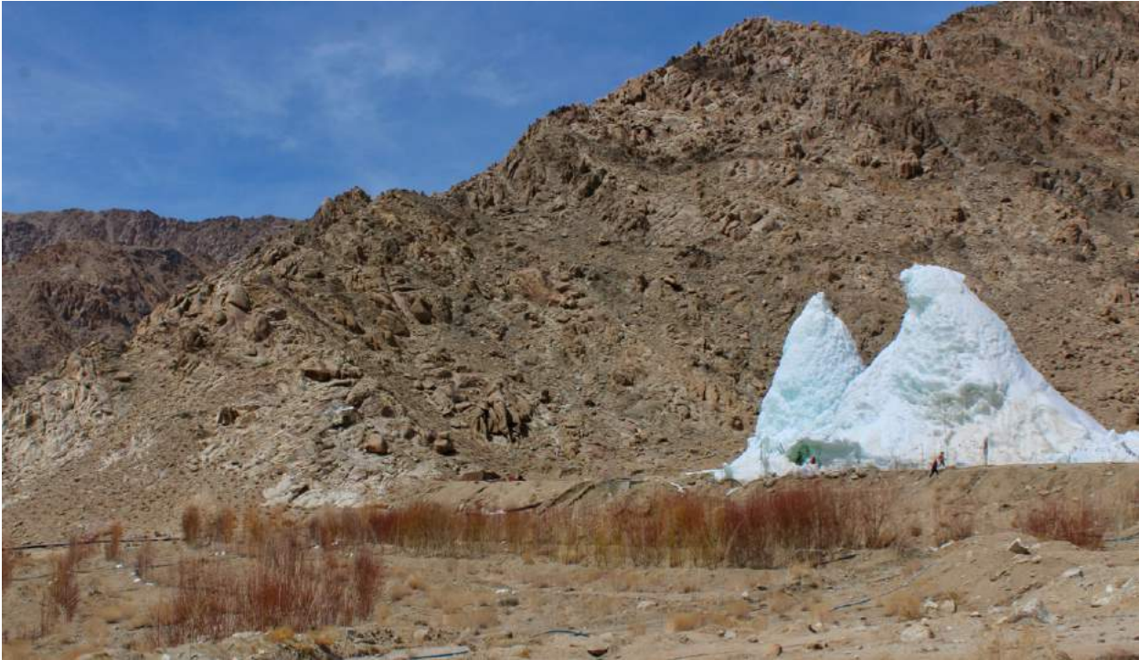
Figure 27. Double ISs sit above a plantation of 5,000 trees owned by the monastery that the structures irrigate.
