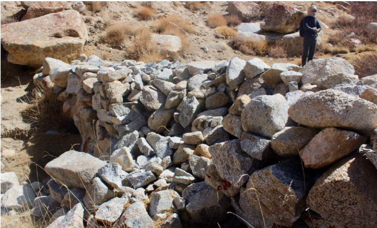
Figure 22. When AGs are made with local stone, like this wall above Phuksey, it is somewhat easier to reuse the same materials to repair the wall rather than having to pay for and import expensive cement.
