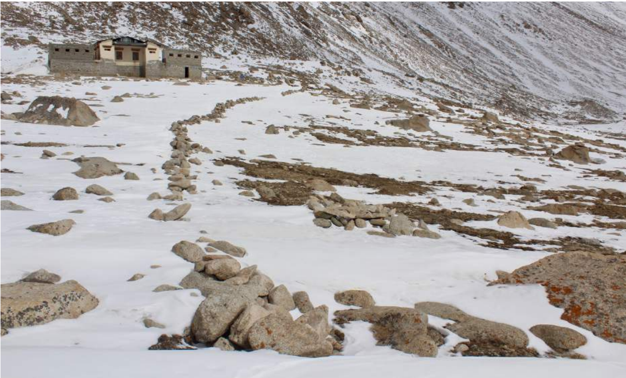
Figure 4. Original kha gags or 'snow block' walls built by villagers on the top of Changla.
