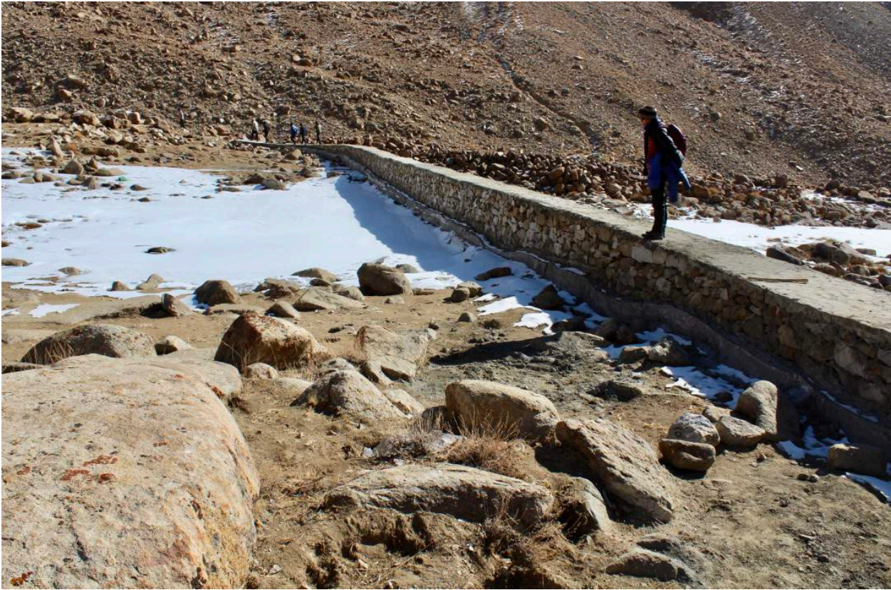
Figure 11. A blocked diversion canal at Likir's AG led to little ice forming behind the lowest wall.
