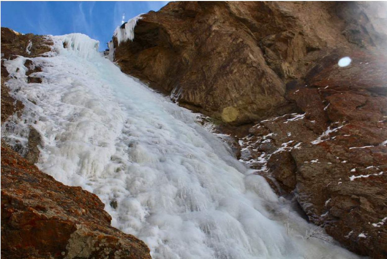
Figure 34. The AIG at Atitse was first built in the winter of 2017-2018. The flexible nature of the plastic pipe enables the position of the water outlet (visible upper left), to be changed every 10 to 15 days to promote greater coverage of the cliff.
