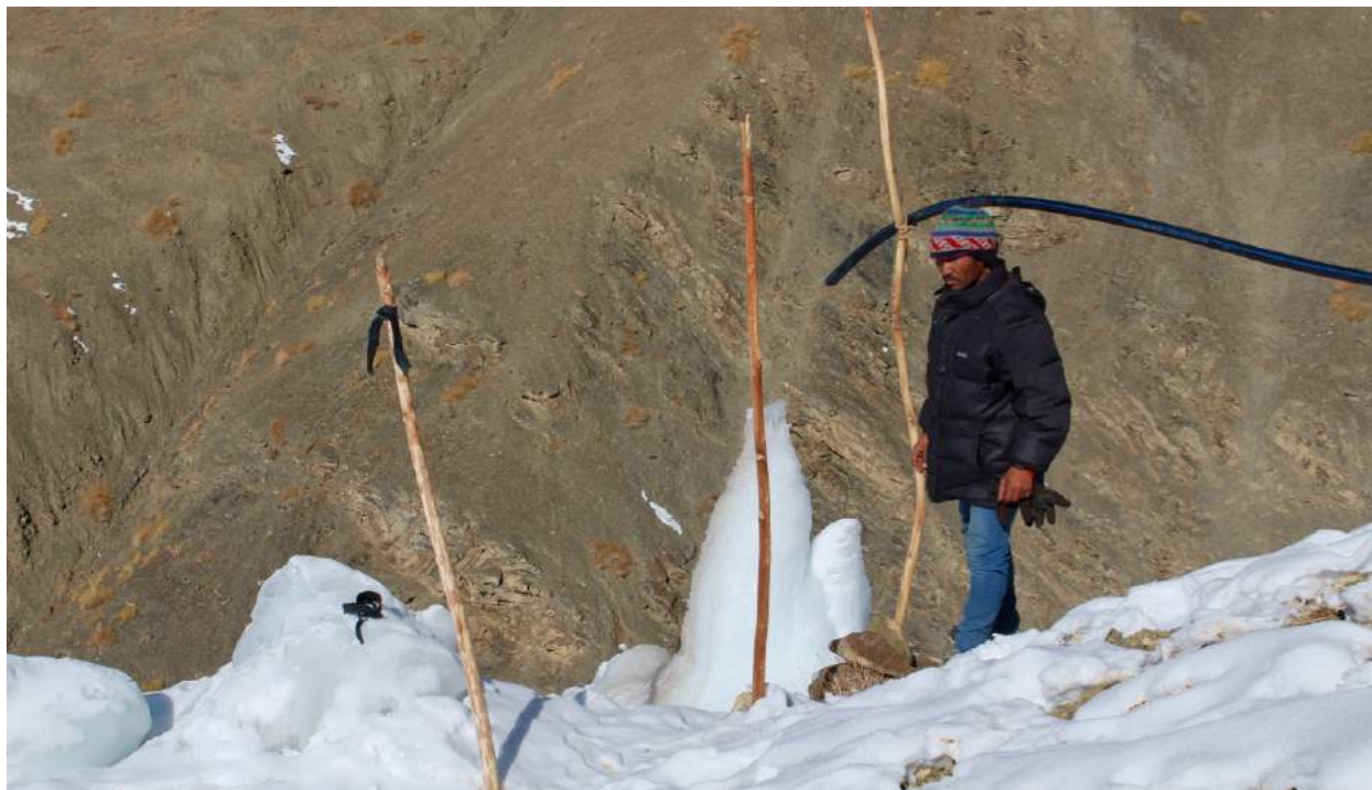
Figure 36. While AIGs have flexibility in their structure, when pipes freeze due to insufficient pressure and low temperatures it can cause a lot of labor for residents. Here a man from Henisku, trekked over 1.5 hours to the site, only to discover the pipe frozen. He must return to dig up several hundred meters of pipe, clear the blockage, and bury it again.
