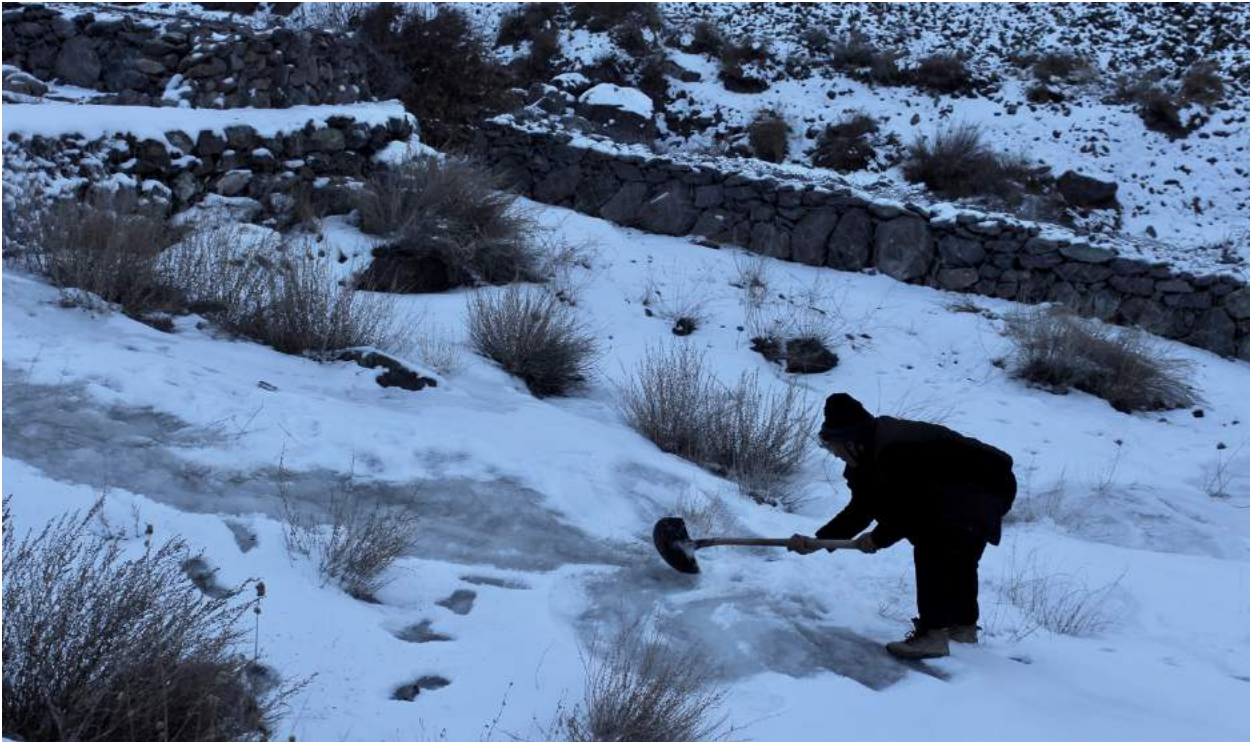
Figure 13. An NGO worker attempts to get water to spread over the surface of the ice reservoir to promote freezing.
