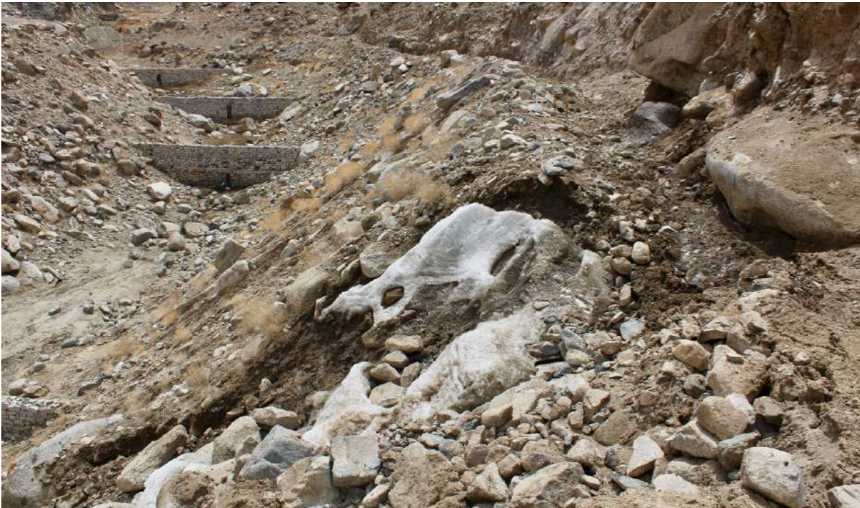
Figure 16. Damage to the canal due as the ground and frozen ice melted on the hillside, saturating the loose soil.
