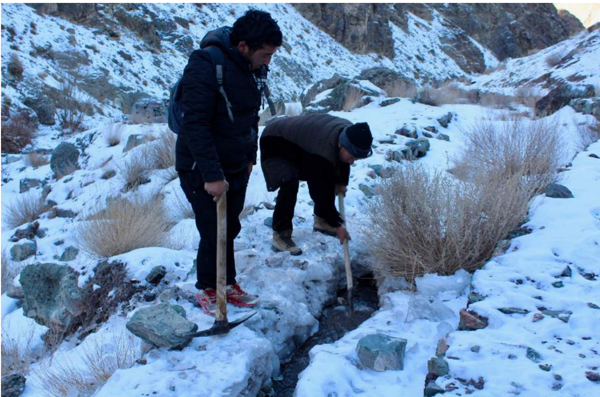
Figure 12. One of the greatest challenges that diversion-style AGs face is the almost daily maintenance required to keep water flowing through the canal to the structure and on top of accumulated ice behind the walls.
