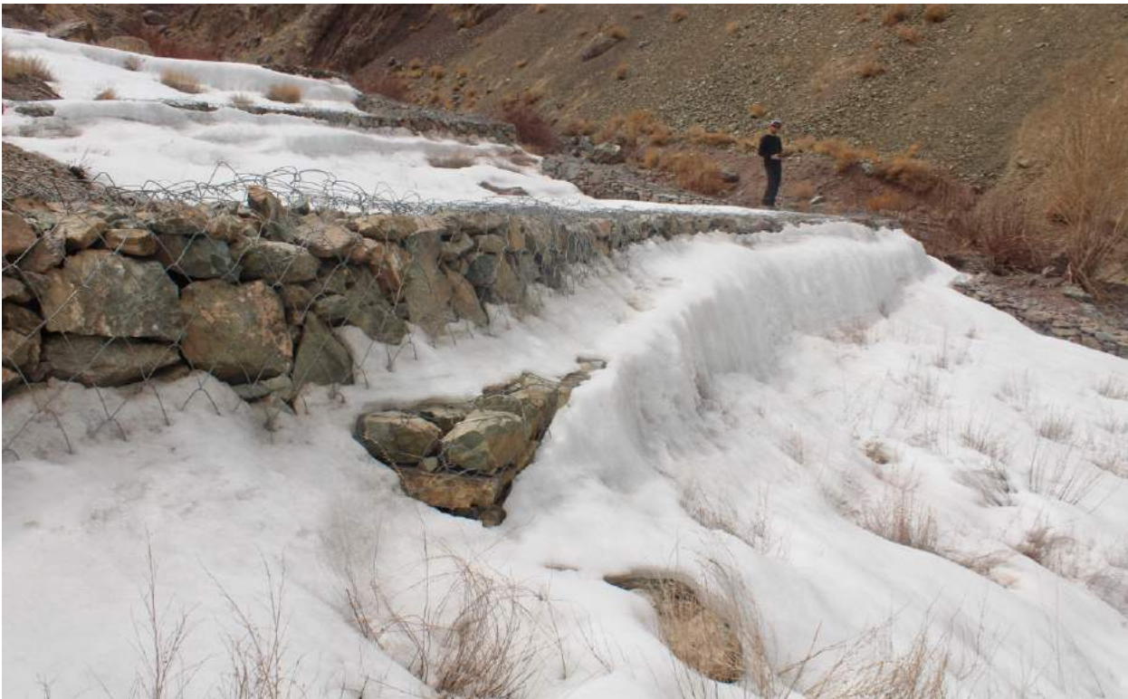
Figure 8. Built in Alchi in 2017 with funds from the Tata Trusts, this is one of a few diversion style AG functional today.
