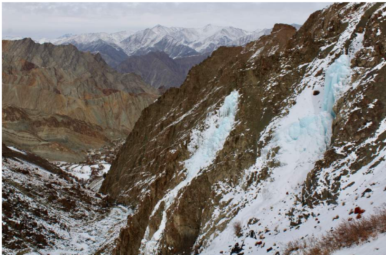
Figure 33. The site of the first AIG above Kuksho was chosen in 2016 by HH Chetsang Rinpoche in consultation with monks from Lamayuru Monastery and villagers. The shaded slopes of this ravine receive little sunlight in the winter, making it an ideal location for ice formation. Nearly 100 meters tall, this structure depends on spring water piped one kilometer from late October to March when temperatures remain below freezing.
