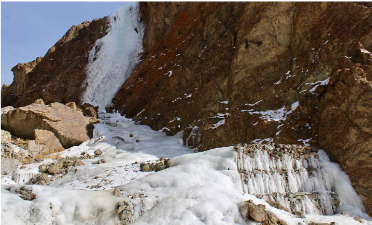
Figure 38. AIGs have great potential to be combined with other AGs like in-stream ones. Here, Atitse's AIG was built above a series of dilapidated rock walls. Even in their current state of disrepair, these walls greatly increased ice accumulation in the valley below and residents are hoping to build more walls in the future.
