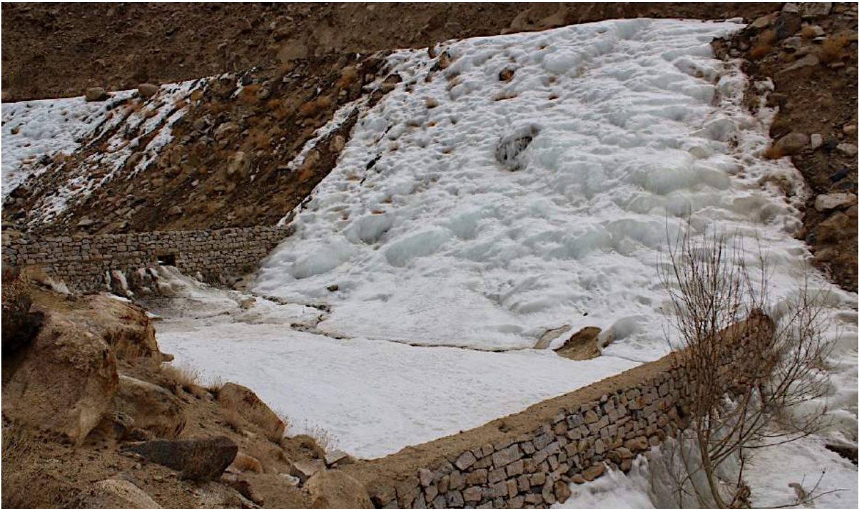
Figure 14. Modified diversion-style AG at Nang where water flows over the edge of a canal and into walled reservoirs.
