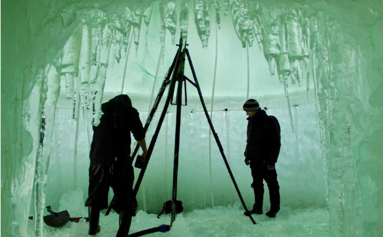
Figure 31. Inside the dome of an IS, new sections of vertical pipe are added to increase its height. Issues with frozen and bent pipes, however, are also some of the greatest challenges to the project and require a full-time team working all winter.
