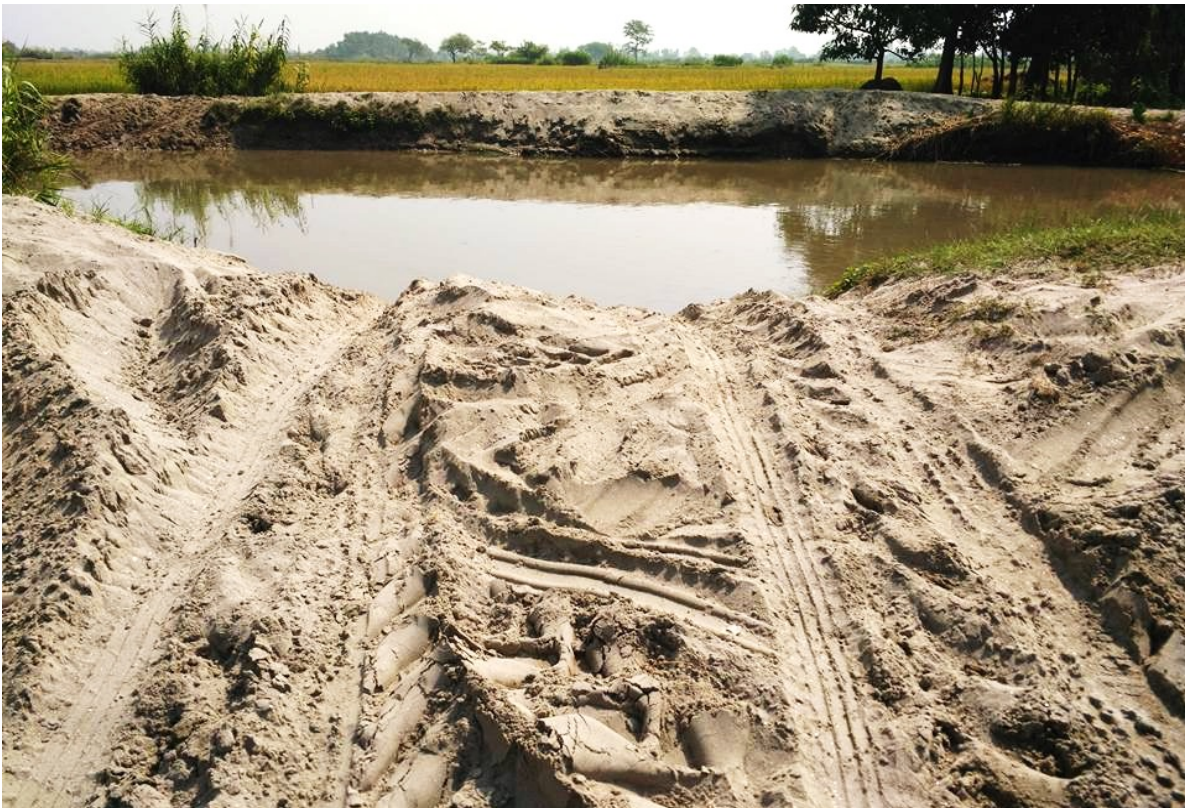
Figure 20. Heaps of sand line the banks of the Budhi Kulo ’s branch canals, overwhelming farmers who have nowhere left to haul it. Due to the amount of sand dumped on adjacent roadways, several can no longer be used.
