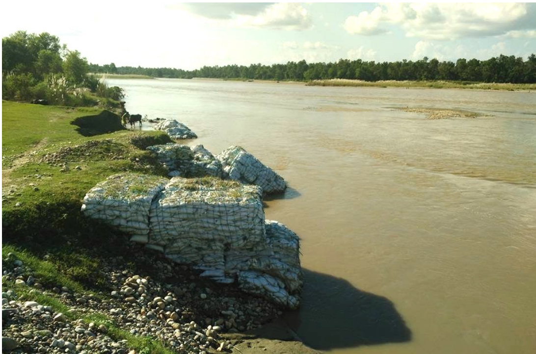
Figure 32. A temporary embankment built to protect an active construction site upriver slumps into the Karnali River as monsoonal floods undercut the structure. While gabion structures are stronger than these sandbag and rope spurs a similar process can occur as the wire rusts and weakens.
