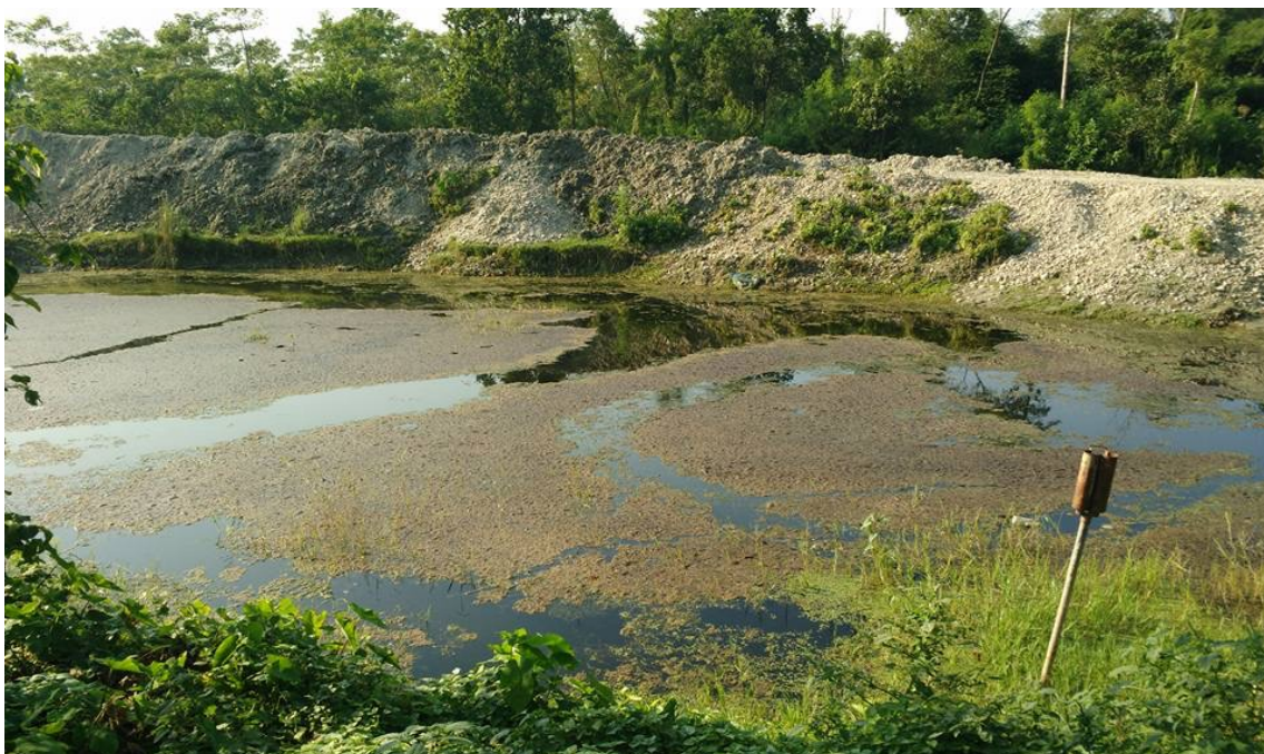
Figure 21. A partially-completed embankment of the Karnali River Training Project. The remains of a water pump are still visible in the foreground where a community of bonded laborers lived until they were displaced by chronic waterlogging associated with the structure.
