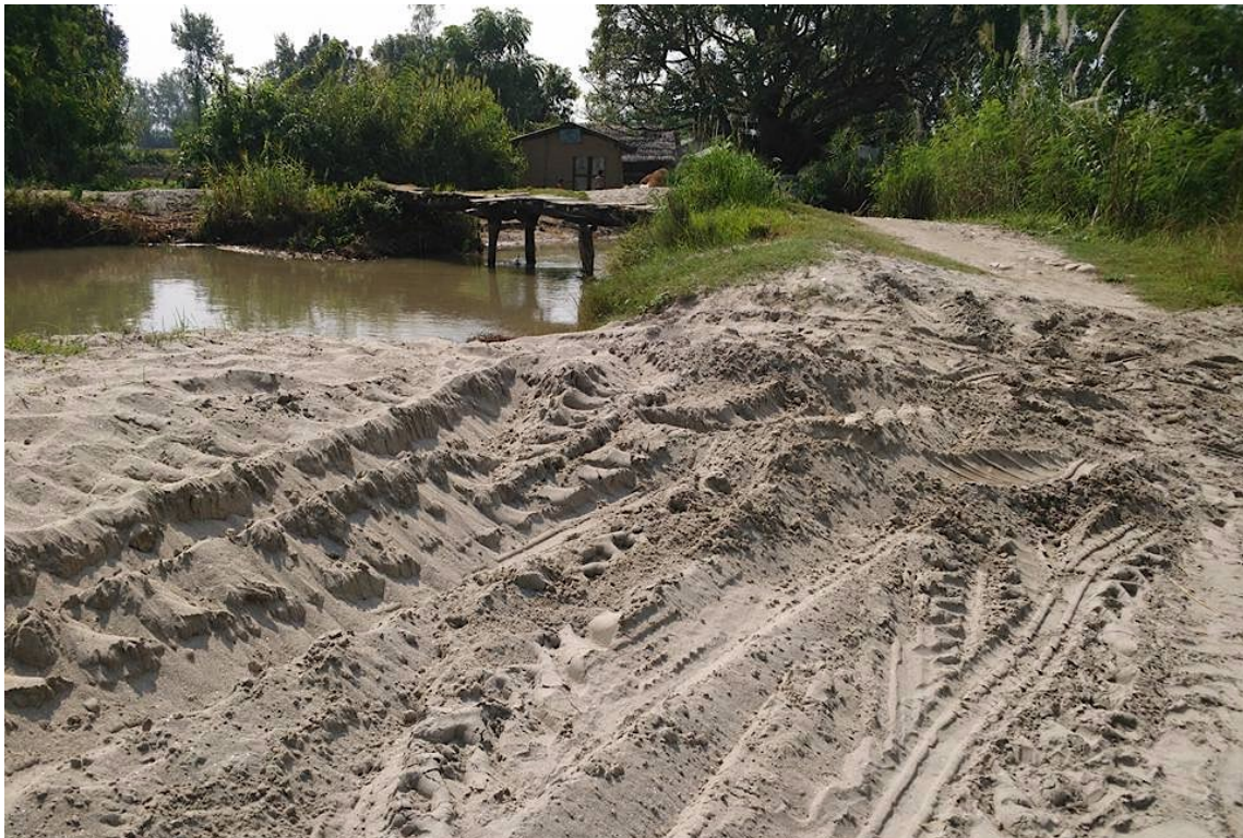
Figure 15. Excavated sand piled along a branch canal of the Budhi Kulo .
