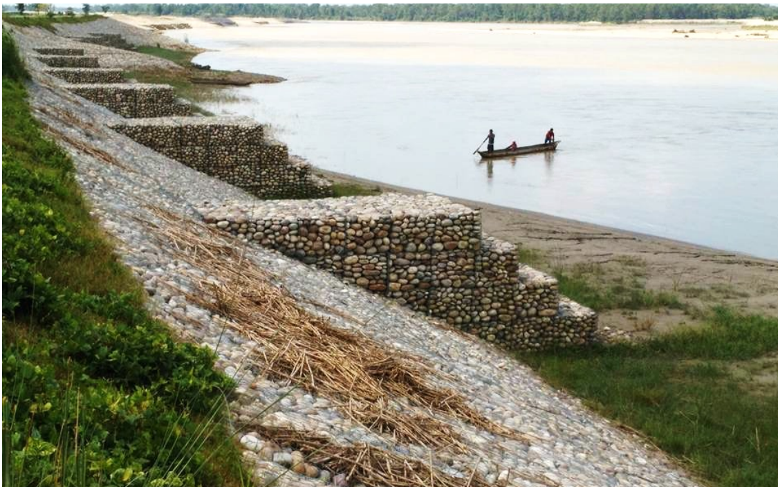
Figure 27. This embankment was built during the first year of the Rajapur Irrigation Project to deflect the Karnali River back toward Thikapur, directly across the river and from where this canoe ferry is coming.
