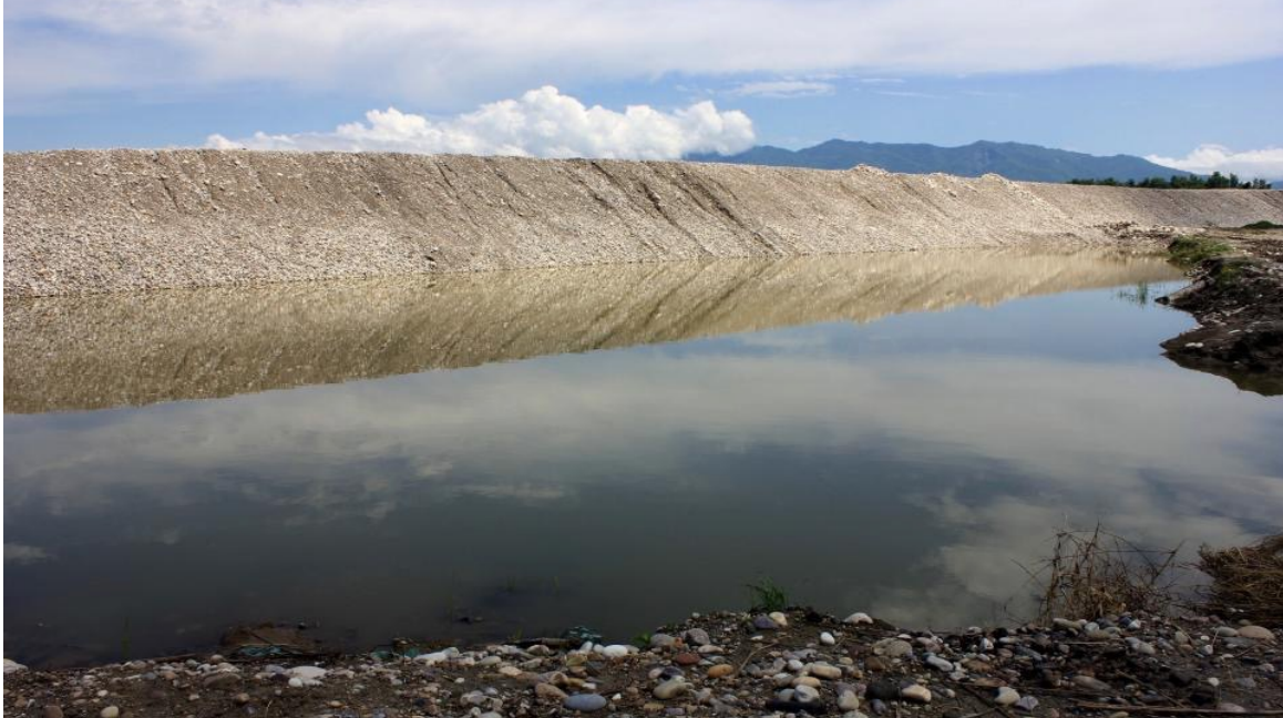
Figure 30. Embankments prevent drainage, creating massive waterlogged areas like this pond in the foreground particularly during the months of monsoon.
