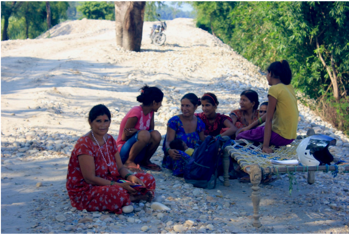
Figure 5. Focus group with women who now live at the foot of an embankment actively being constructed on the island of Rajapur as part of the Karnali River Training Project.
