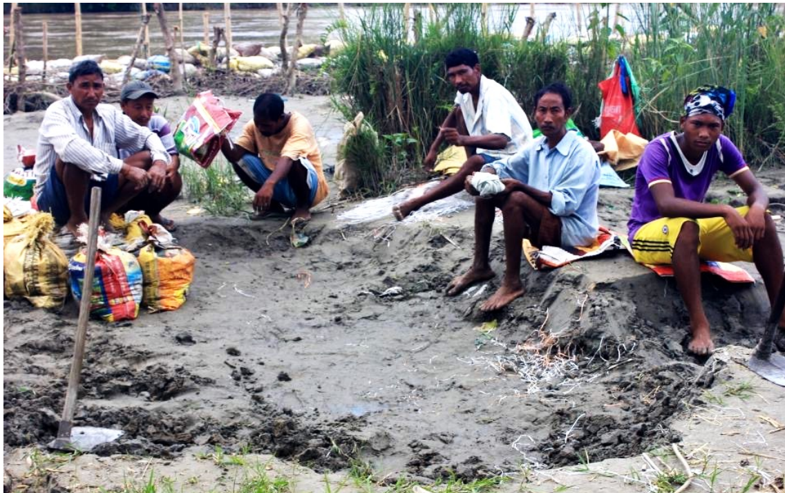
Figure 13. Laborers take a break from filling sandbags to reinforce the emergency structure illustrated above. They are using the half meter of sand that was washed into their rice paddies where the Budhi Kulo breached its banks since this debris will have to be scraped from the the fields if the farmers have any hope of reclaiming soil fertility. As the bed of the Budhi Kulo rises due to rapid sedimentation, cases like this of destructive sand casting occur more frequently along the island's irrigation canals.
