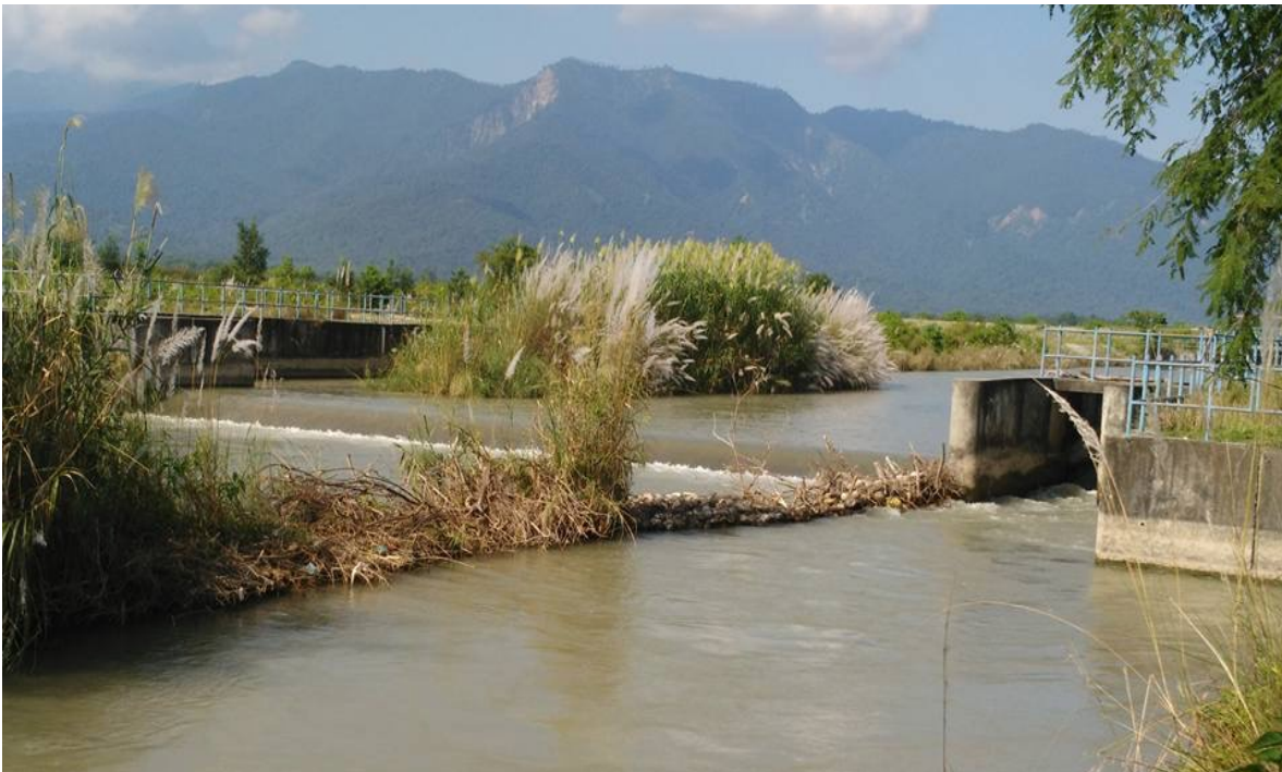
Figure 18. This Tharu-style bandh whua was built as an extension on top of a concrete intake in order to repurpose existing infrastructure that had been built during the Rajapur Irrigation Project. This hybrid bandh whua -concrete structure is being used to direct water into a newly dug canal that was built by farmers to replace one of the concrete intakes that had to be abandoned due to sedimentation.
